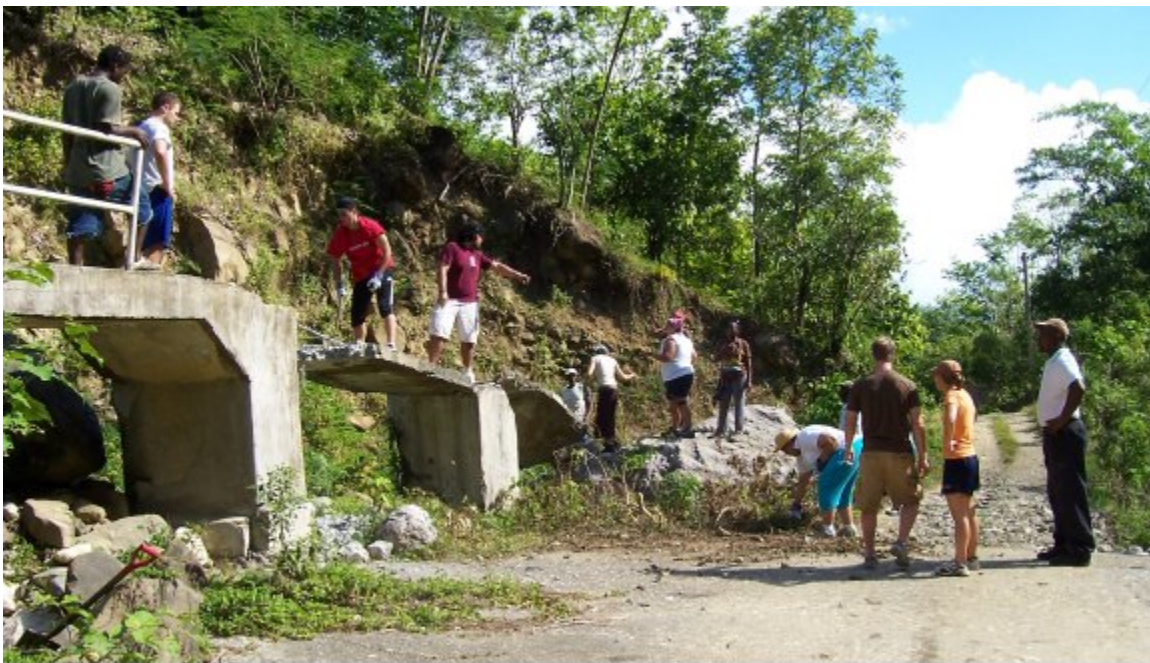
St. Lawrence students begin work re-building a bridge in Jamaica
